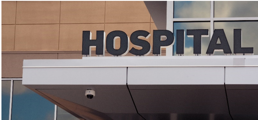
Figure 1155-12: Example of a canopy sign
