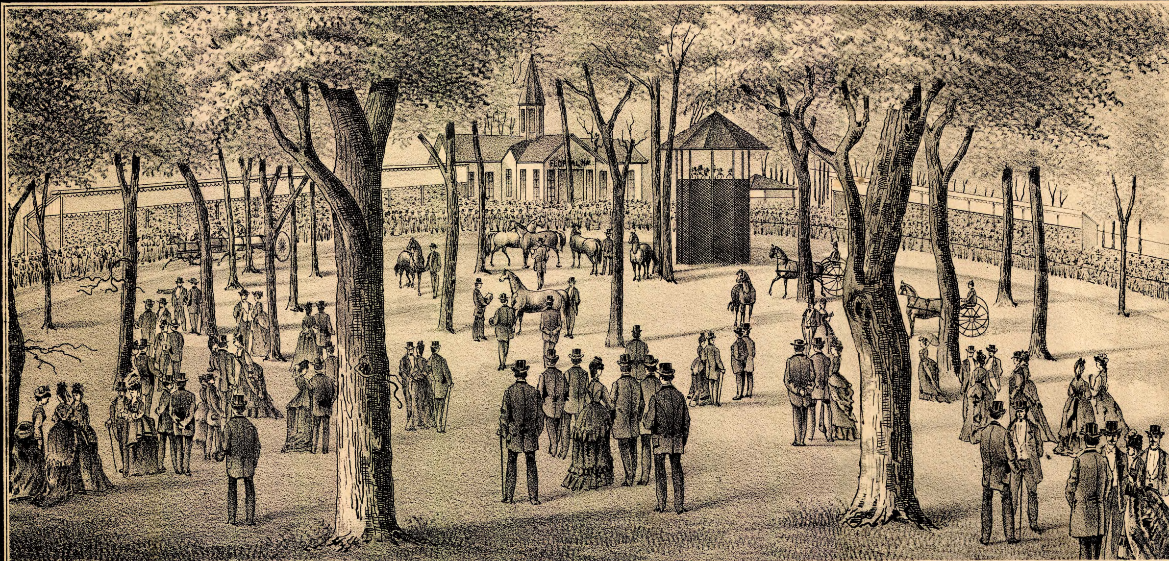
SOUTH VIEW OF EXPOSITION BUILDING & AMPHITHEATRES.
